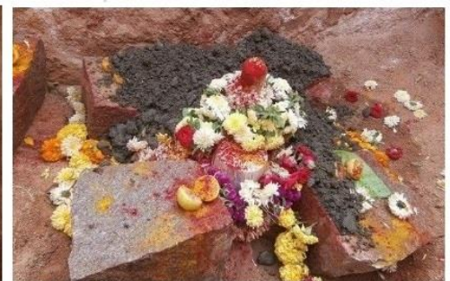
After the pooja - concrete is poured
