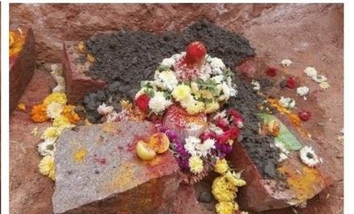
After the pooja - concrete is poured
